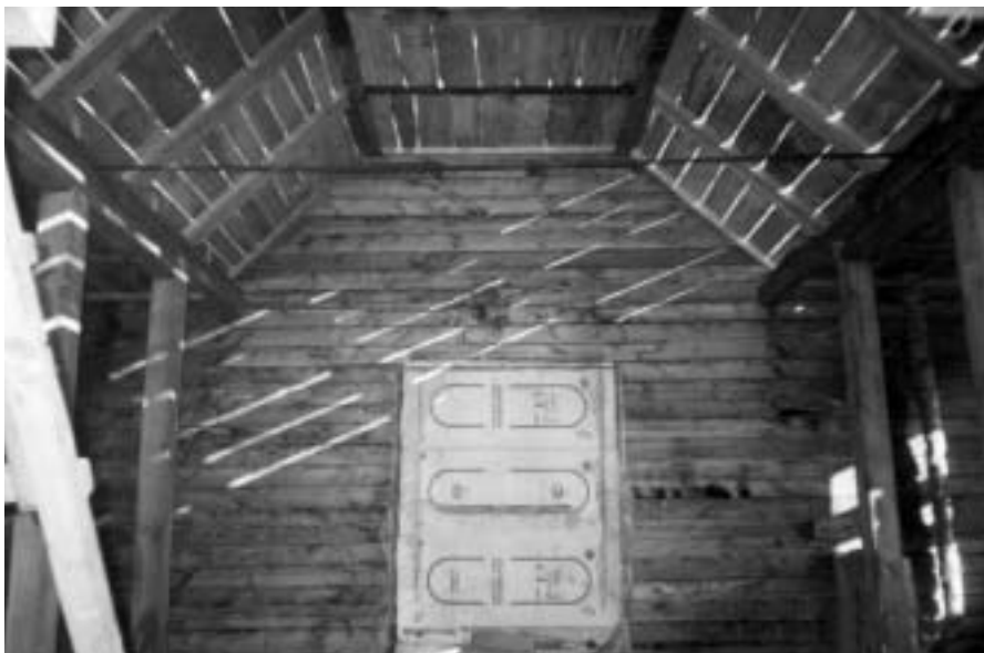
Unfinished nave of St. Nicholas Church.
