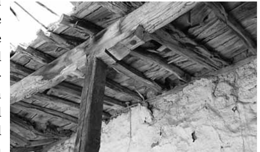
Use of branches and reeds in construction, from the scarcity of wood in the area.
